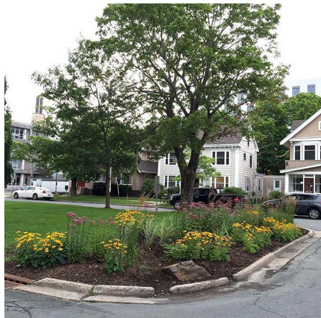
Figure 5: Institutional Rain Garden with a central drainage channel, curb cuts to allow road drainage, and perennial plantings.
