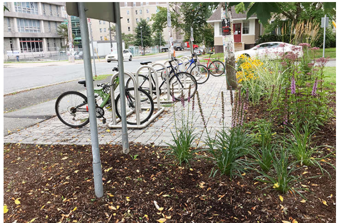
Figure 4: Institutional Rain Garden beside a permeable paver bike parking pad.
