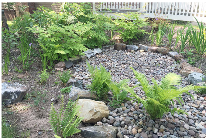
Figure 1: Residential-Scale Rain Garden with a planted soil berm and deep gravel drainage bed.
