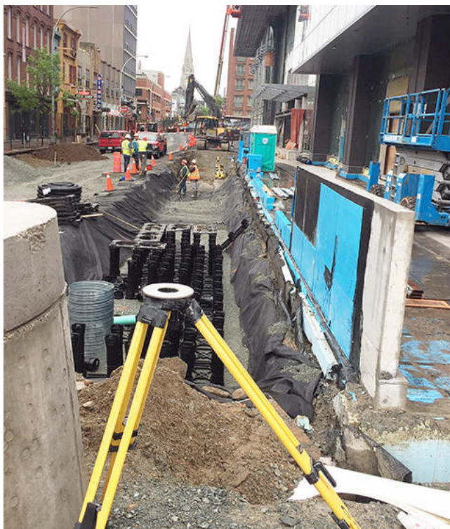
Figure 2: Soil Cells. Highly impervious situations can be engineered to have planted soil cells with backup drains tied into the municipal system. This was the case with the Argyle Street streetscaping project in Halifax,
